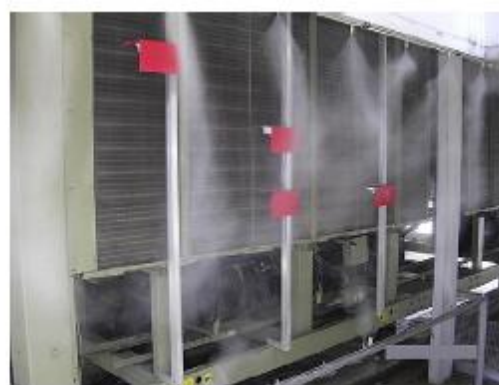
Fig.2.4 . Water mist precooling
